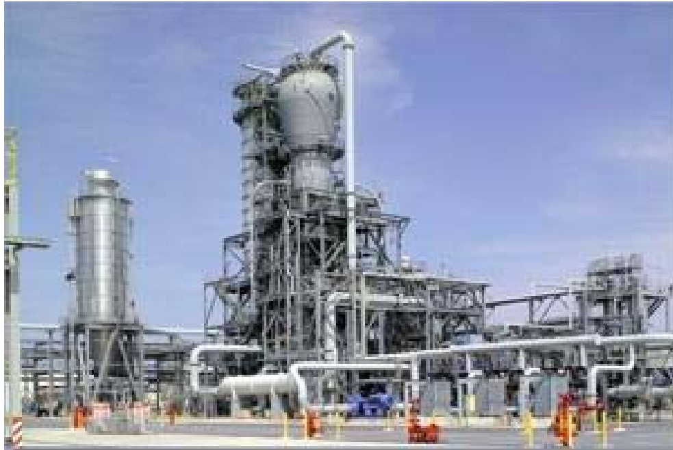
Figure 9: Industrial scale UNIPOL reactor (Univation Technologies, 2004)
