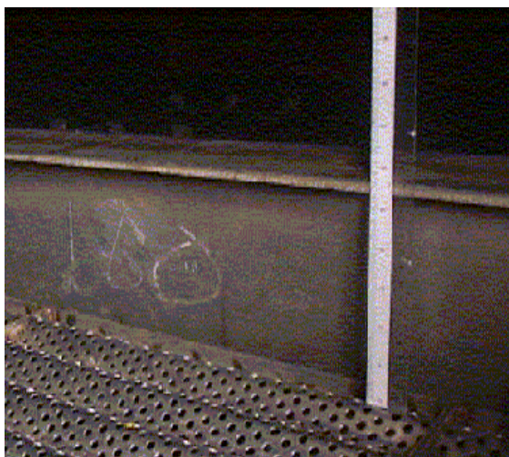
Figure 1: 6" I-beam installed on the tray.
