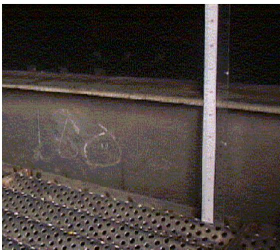
Figure 1: 6" I-beam installed on the tray.
