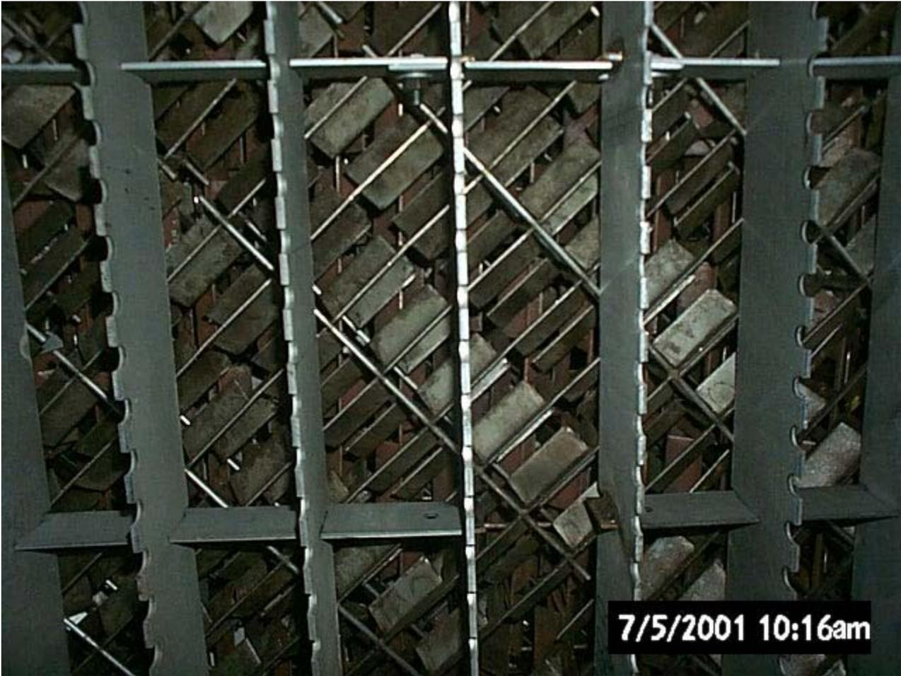
All of the packed beds include a hold-down grid and support plate with beams to meet a 2-PSI uplift specification. The grid is through bolted for extra strength and stability.
