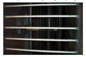
increase the overall cost and complexity of the system. The basic design of an ammonia injection grid is simply a series of perforated pipes connected to a manifold. The cost of this equipment is higher in SNCR than one suited for SCR due to the metallurgy required for high temperatures. Alloys containing chrome, molybdenum and nickel such a Hastelloy and Inconel are typical examples.
